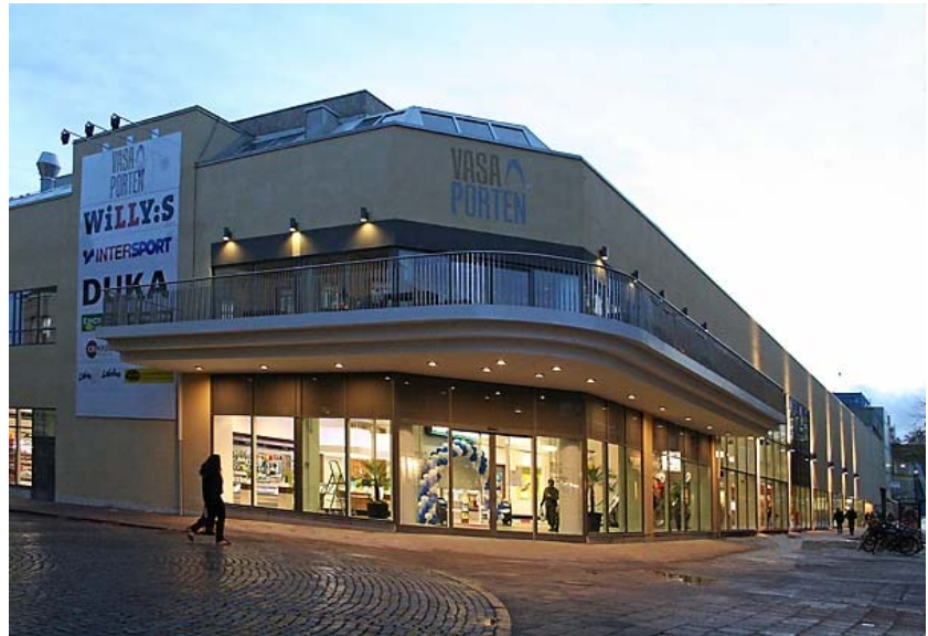
Picture of Vasaporten after the renovations
