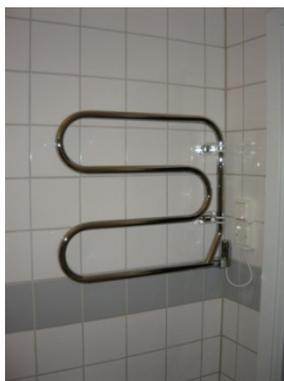
*During construction the existing radiator was removed and replaced with an electric toweldryer as in the Malmö region, this gives the landlord the right to charge a rent of a further 35 kr / month*
